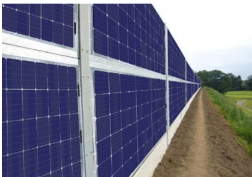
Noise barrier, horizontal Mounting (Modules Size II)
