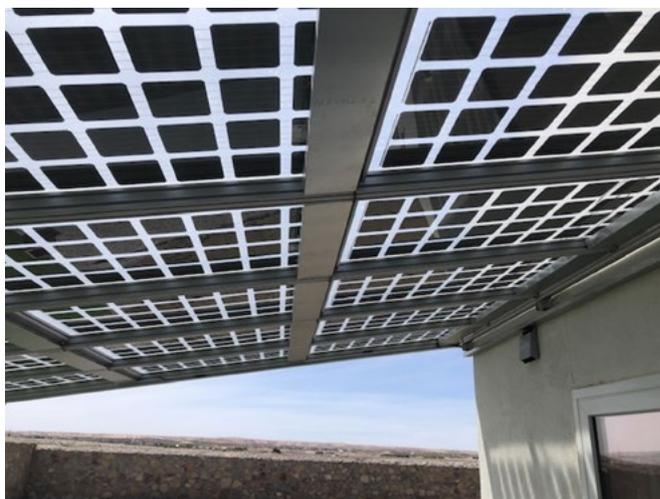
GridParity PV terraces are individually configured from high-quality anodized aluminum as a kit. The transparent double glass modules as well as the waterproof mounting protect the terraces from environmental influences, while they produce energy silently and environmentally friendly. The electricity can be fed into the house grid or into the optionally available battery systems. The integration of charging stations is also possible.
