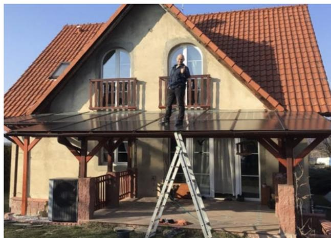
PV terraces offer great potential of solar energy generation. Conventional modules are not suitable for roofing, as they neither transmit light nor meet aesthetic requirements. Therefore, this potential has hardly been used so far. GridParity PV terraces are roofed with transparent PV modules that allow up to 40% light to pass through, thus protecting against direct sunlight on the one hand and creating a cozy atmosphere on the other. For terraces, waterproof installation is crucial.
